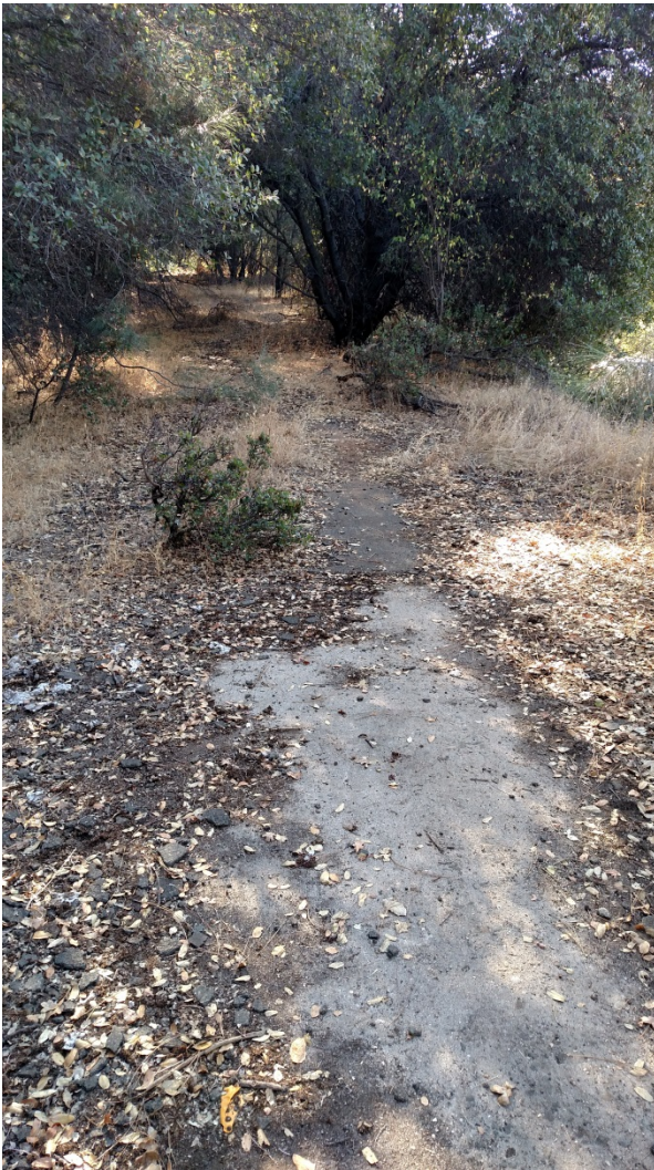
Image 5. Internal view of site; remnants of Lincoln Highway alignment located above Placerville Drive
